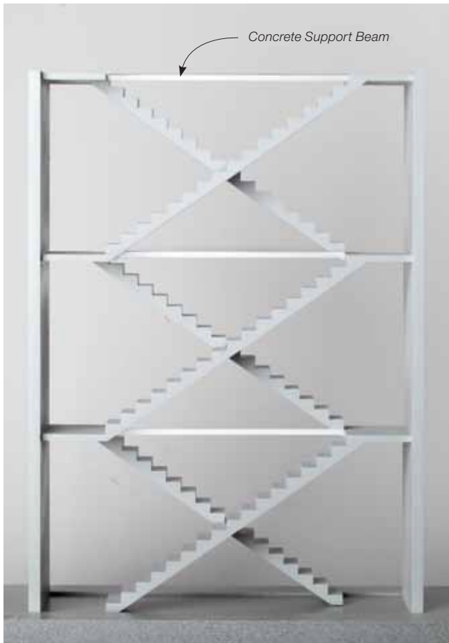
Figure 7 - Scissor Stair Spine Wall Construction
